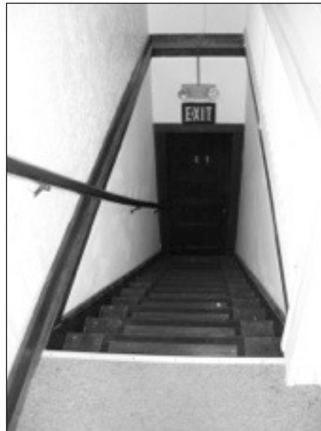
The narrow staircase that leads to the third floor of Fuller Lodge.
